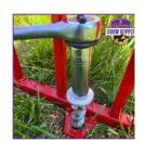
STEP 04: Secure Show Prep Pen to the ground, in 2 places, with the supplied earth anchors. Use a ¾" wrench or ratchet+socket.
